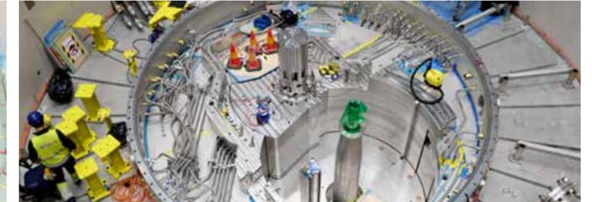
**Target Monolith:** All the neutron beam port inserts and neutron beam windows were installed and successfully leak tested under vacuum. The inner shielding, target wheel and shaft and the moderator-reflector system were installed after remediation of the inner shielding cooling channels for cleanliness and weld/piping material integrity and an endurance test of the target wheel rotation in the Target mock up and test stand.
